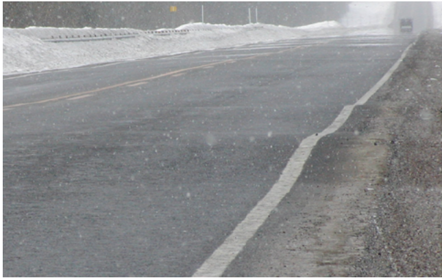
This pavement is lifted by as much as 20 cm.
