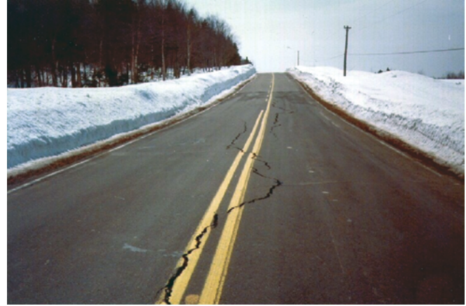
Longitudinal cracking, as depicted in Figure 2
