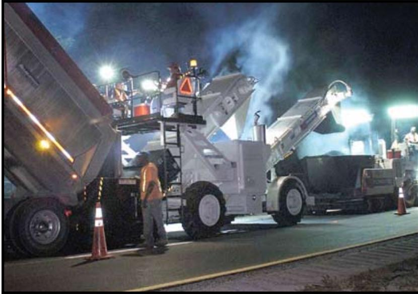
The MTV-1000D material transfer vehicle, like the Shuttle Buggy® models, is capable of transferring while reblending paving material to allow for continuous in-line paving. The patented, offset gravity transfer provides reblending of asphalt materials just before they are delivered to the paver, eliminating truck-end segregation. With an optional windrow attachment, the MTV-1000D can pick up material from a windrow and transfer it to the paver.
