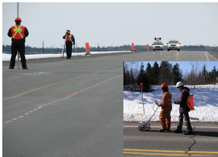
Figure 1: Measurement of frost heaves (rod and level and portable profilometer)
