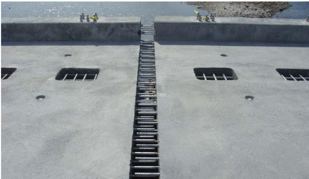
Figure 8 – Joint transversal
