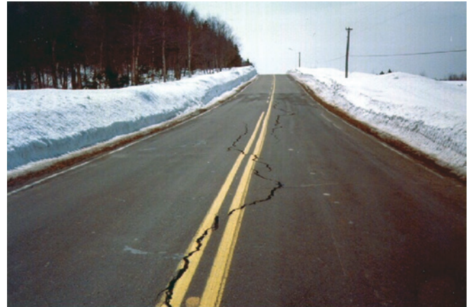
Longitudinal cracking, as depicted in Figure 2
