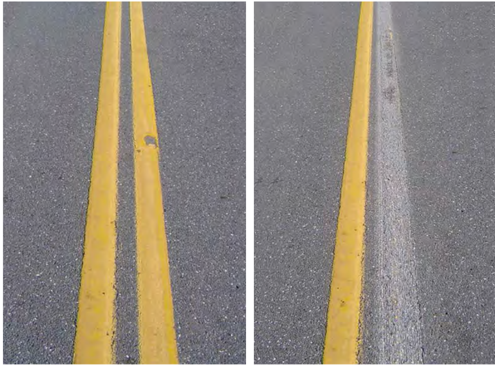
Figure 68 – Example of removal work by mechanical abrasion (before and after)
