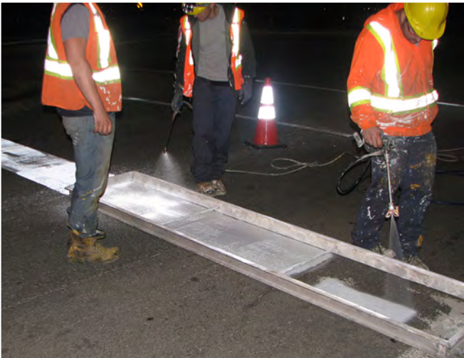
Figure 4 – Application of special marking using a pressure gun and stencil
