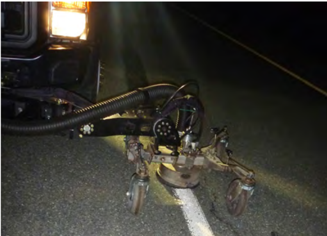
Figure 69 – Examples of removal with high-pressure water blasting
