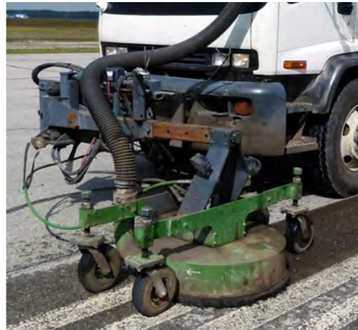
Figure 69 – Examples of removal with high-pressure water blasting
