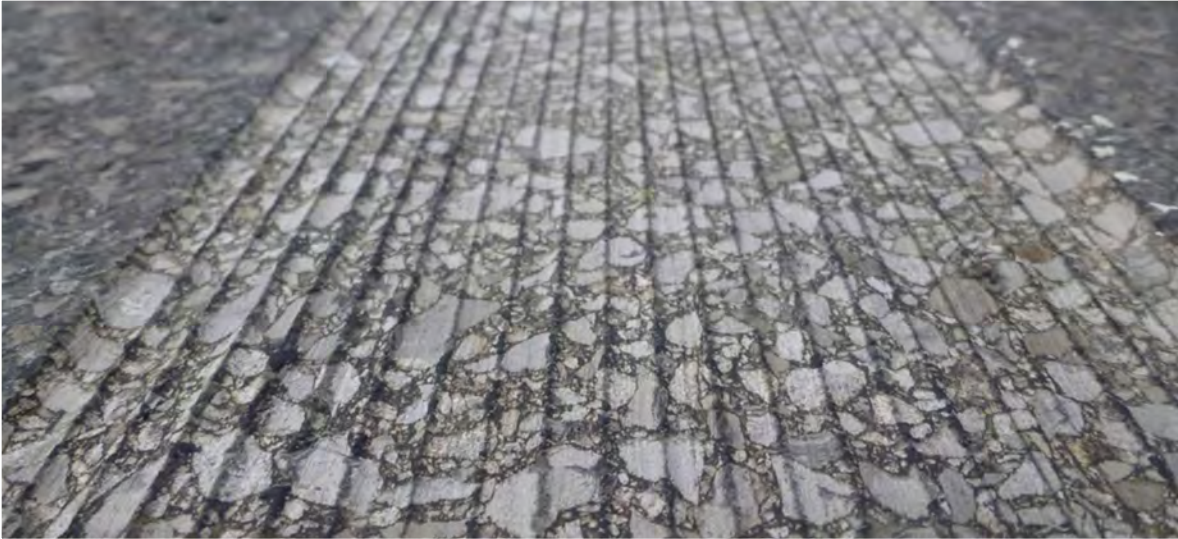
Figure 33 – Example of an irregular finish groove with ridges (non-compliant)
