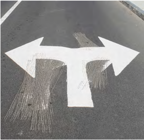
Figure 80 – Example of non-compliant removal using a grinder
