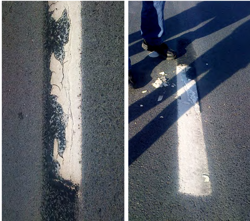
Figure 62 – Application of an epoxy resin-based material on a product that has not hardened
