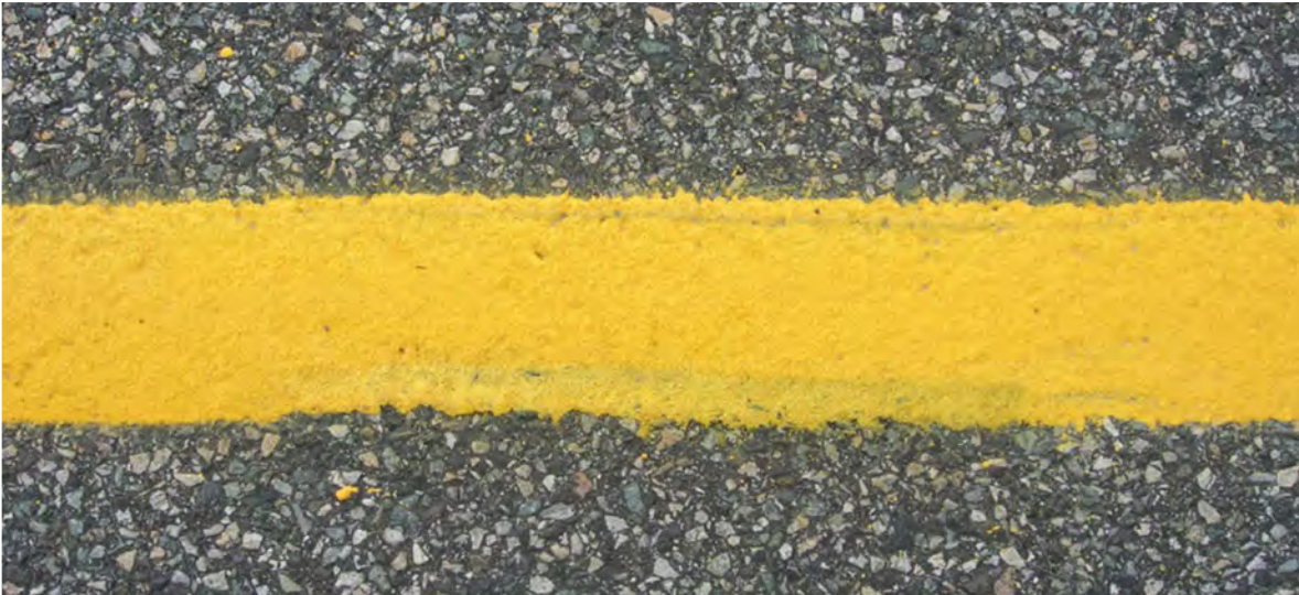
Figure 53 – Marking line immediately after the work
