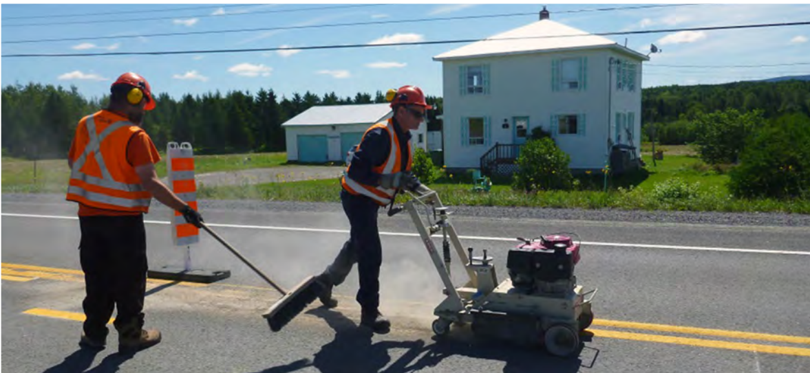
Figure 66 – Example of hand removal unit
