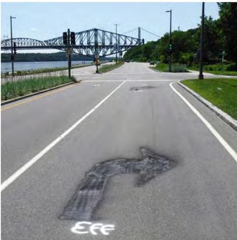
Figure 78 – Example of masking with black paint, daytime (non-compliant)
