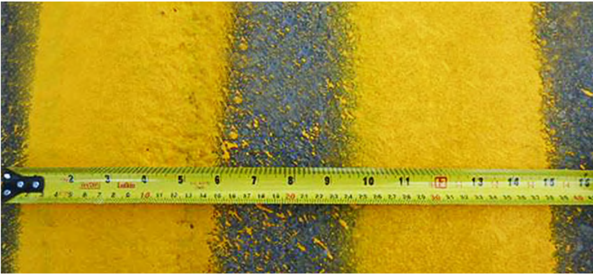
Figure 21 – Example of double solid lines that are too wide and not spaced far enough apart
