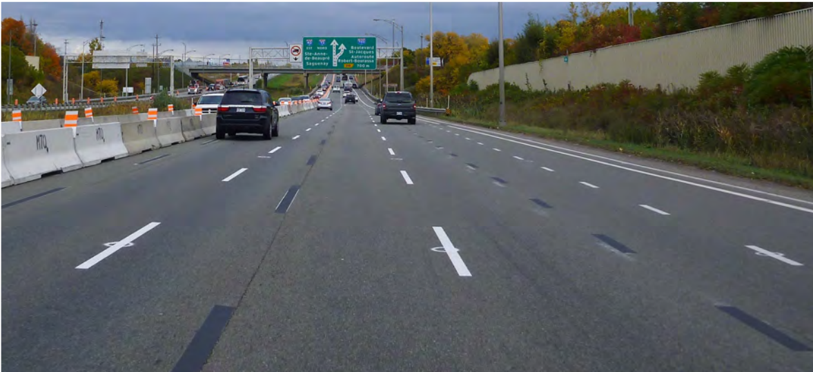
Figure 76 – Proper use of black pavement marking tapes
