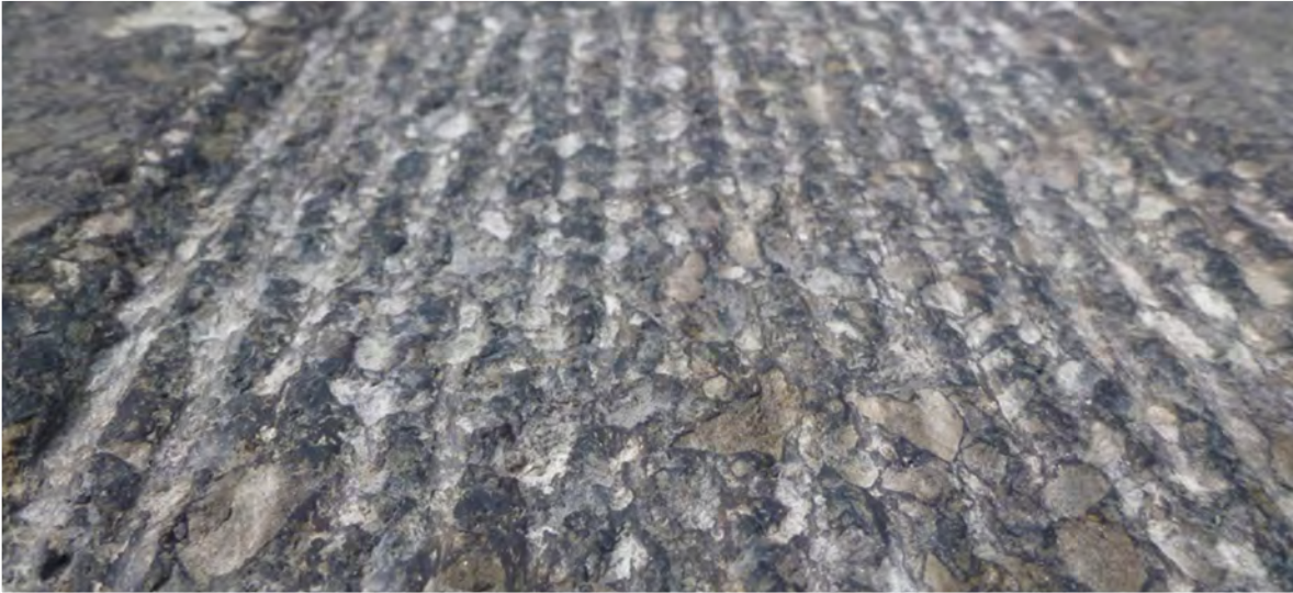
Figure 34 – Example of a rough finish groove (non-compliant)
