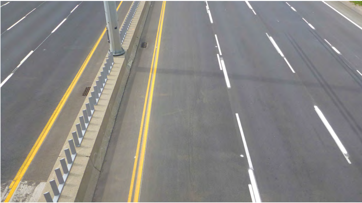
Figure 9 – Example of misalignment of pre-marking and inlaid marking
