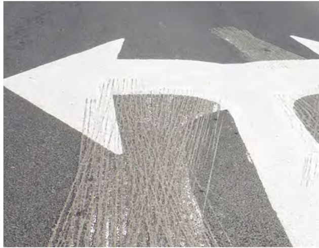
Figure 81 – Example of non-compliant removal using a grinder (close-up)
