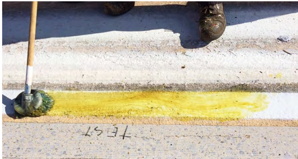
Figure 82 – Example of removal with a chemical stripper (non-compliant)
