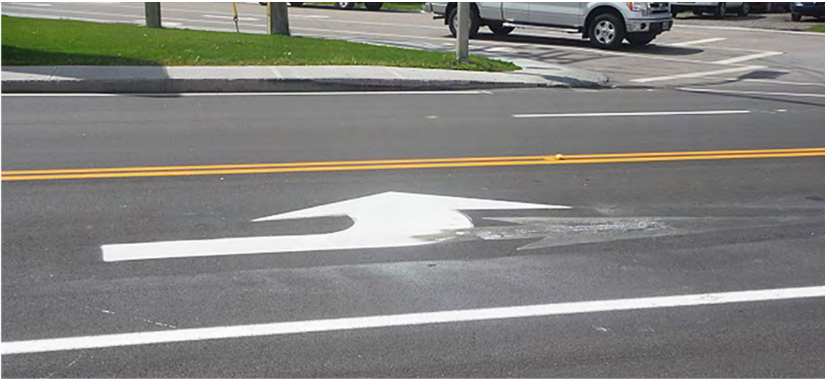
Figure 58 – Disappearance of a portion of a symbol (example 1)
