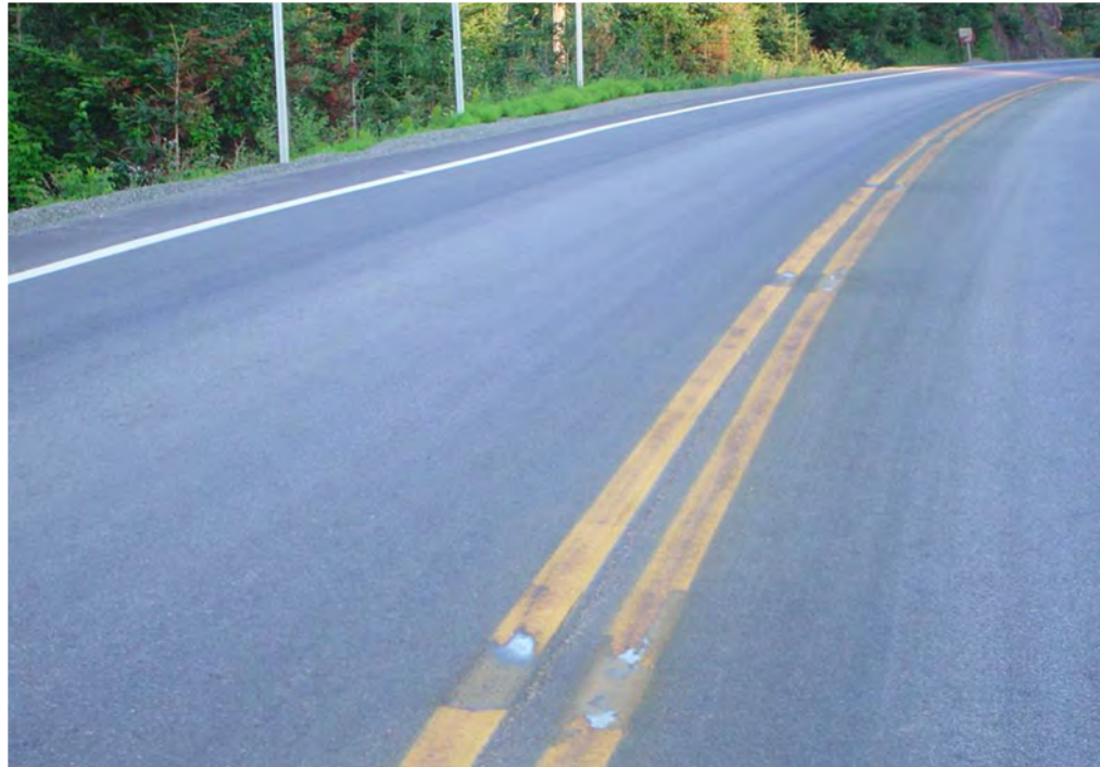
Figure 55 – Recurring problem of poor mixing (pump stroke of the striping truck)
