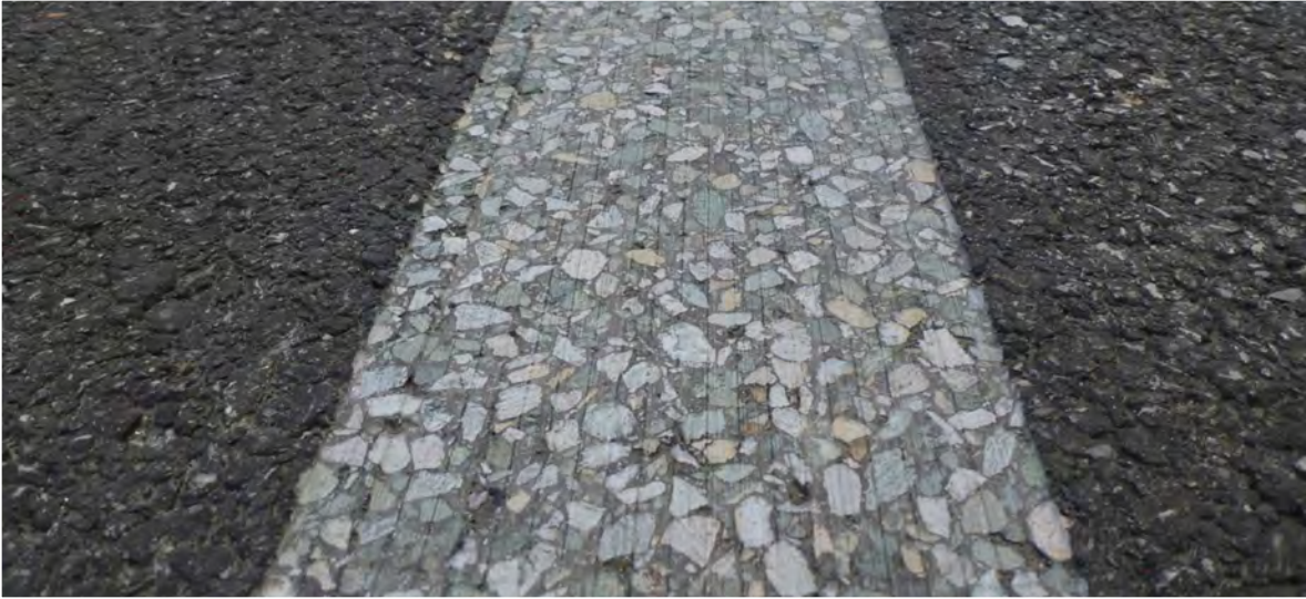
Figure 31 – Example of compliant smooth-finish groove
