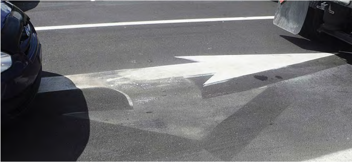
Figure 59 – Disappearance of a portion of a symbol (example 2)
