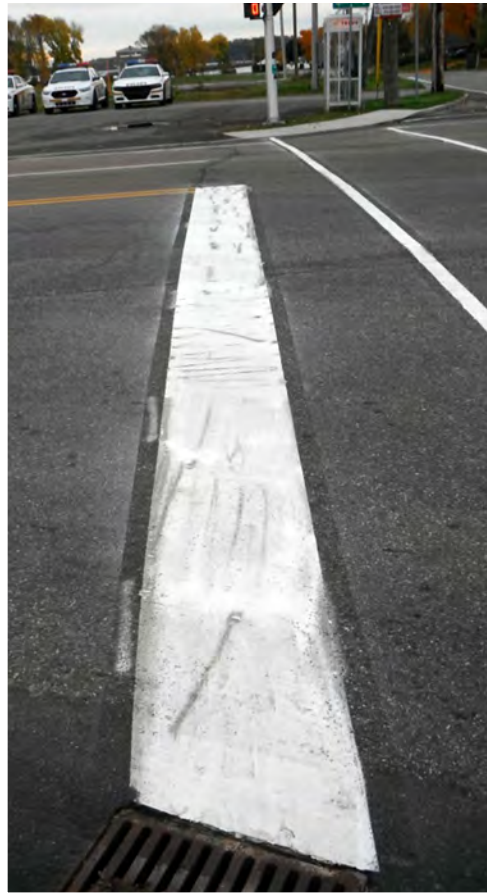
Figure 57 – Darkening of a stop line (example 2)
