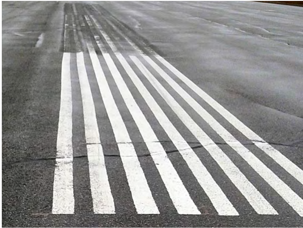
Figure 74 – Premature degradation of the marking occurring directly on the area removed using high-pressure water blasting (top of the photo)
