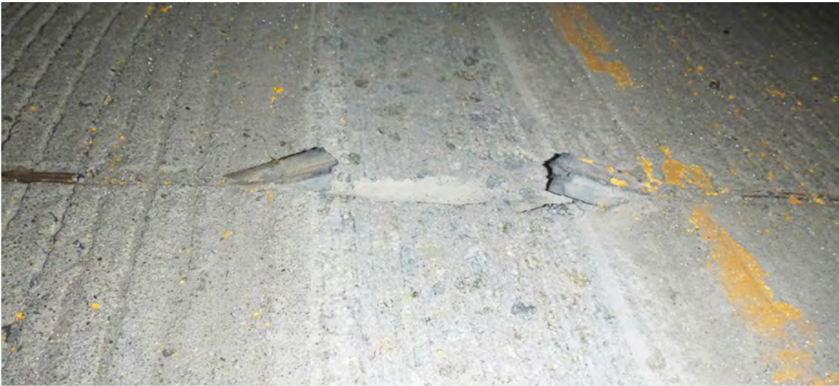
Figure 44 – Tearing off of pre-moulded sealant
